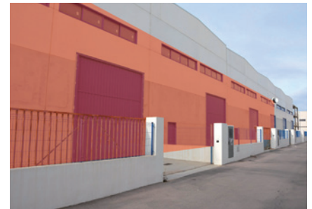
Wall protection (outdoor) at Warehouse
